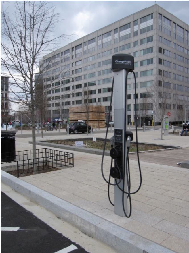
Figure 14. Dual level 2 charging station at Canal Park
